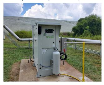
The PowerGen LFG features an auto-tuning fuel train, enabling smooth operation on the fluctuating compositions and low methane levels typical of landfill gas, down to 20%.
