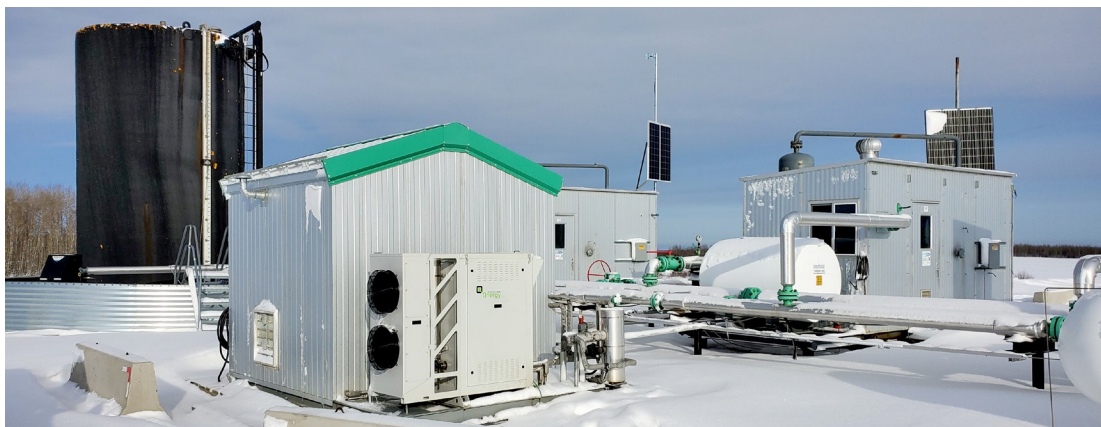
Figure 4. Full-skid deployment during winter providing 500 scfh of instrument air, 1,200 Watt of power and 40,000 Btu/h of heat
