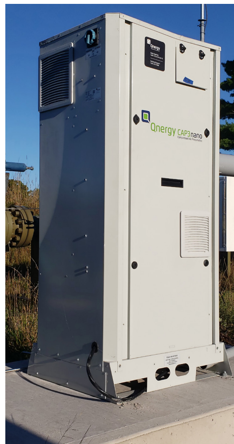
Figure 12. Continuous improvement, relentless innovation. Depicted is a recent deployment of a beta version of the new Qnergy CAP3nano which produces 3 scfm instrument air at 140 psi. As noted in Table 1 , there are many small wellpads in existence which are often deemed too small to warrant capital expenditures to solve methane venting. Qnergy continues to work with clients to create products to fit power, compressed air needs as well as environmental operating challenges such as operating in temperature ranges from -40F to 140F in the most remote sites-eliminating the need for onsite maintenance and human intervention for years of continuous operation. Our goal is to eliminate operational challenges to methane abatement through wellpad automation accomplished at the lowest cost to abate value in the industry.
