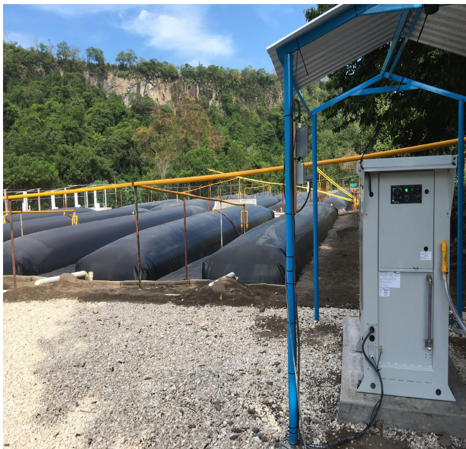
Figure 11. Qnergy and Sistema.bio collaboration on pig farm anaerobic digestion. Foreground shows Qnergy PowerGen unit creating up to 5.6kW of electricity from high H 2 S containing raw methane gas derived from anaerobic digestion of pig manure (background, black bags). On farm generation of useful heat and power creates a circular economy from manure and crop waste when combined with anaerobic digestion technology as well as potential carbon credits.
